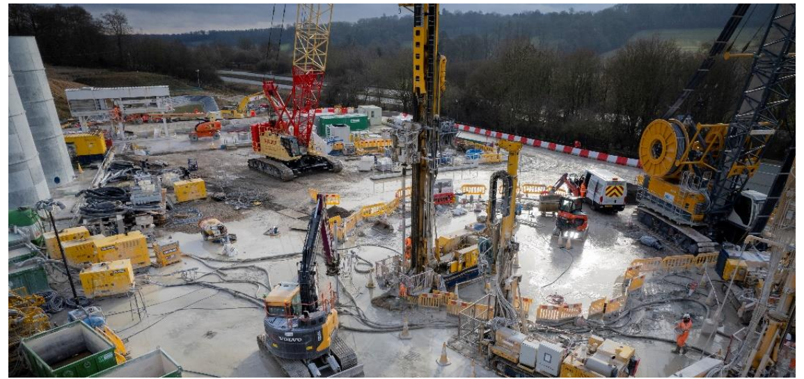
Chalfont St Peter Ground Treatment
