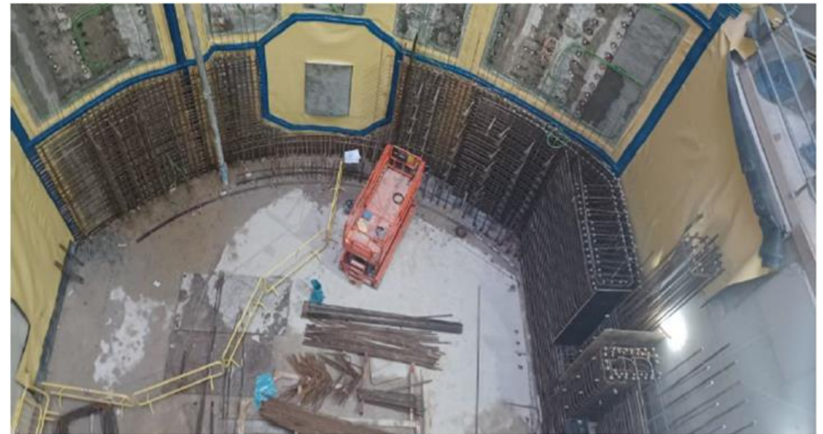
Chalfont St Peter Collar Installation
